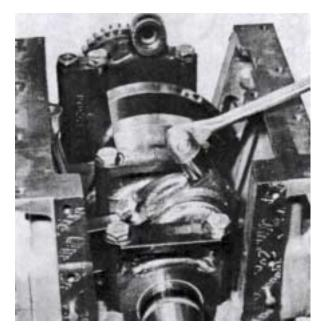
Remove the 4 bolts holding the timing gear casing. The casing also sits on guides. Carefully lever all round and remove the casing.
